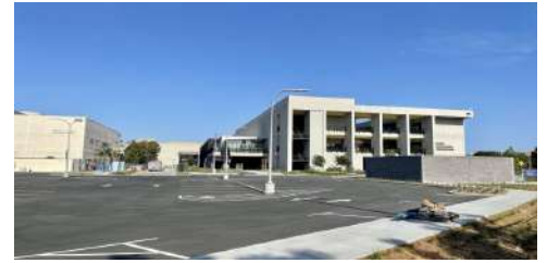
New Science, Engineering and Mathematics Building [Construction]
