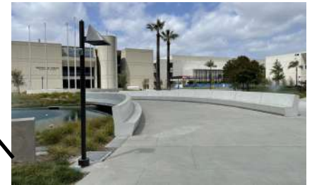
Veterans' Memorial Bridge, Plaza, & Tribute Garden [Close-out]
