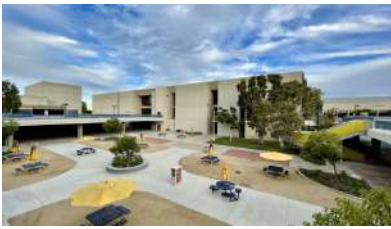
Fine Arts Building Renovation [Design - Construction Documents]
