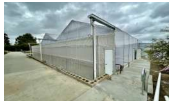
Greenhouse Replacement [Close-out]
