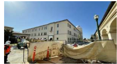
New Instructional Building [Construction]
