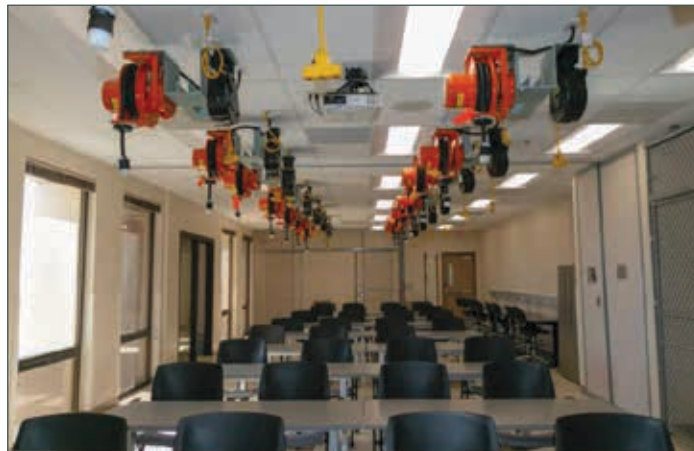
5th Floor Electrical Program Lab
